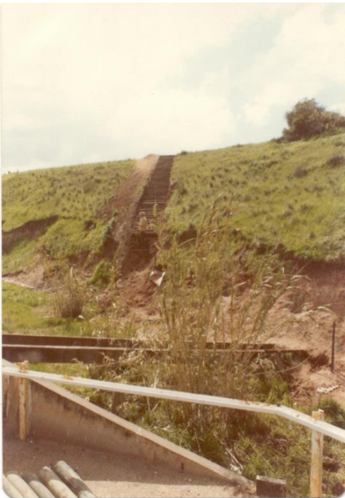
1978 same bank – walkway construction underway. Courtesy of Coast Protection Board
