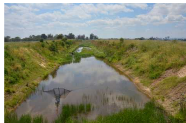
Much of the lower reach of the Harvey River has been channelised. Note the fyke net positioned facing downstream, to capture fish that were moving upstream
