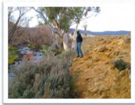
Photo 3. Fencing is often the most important first step in repairing and protecting stream bank vegetation. This fence was positioned too far down the stream bank to provide adequate protection from livestock.
