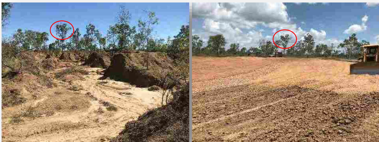
Plate 1 Before and after remediation works at the Treatment 1 site
