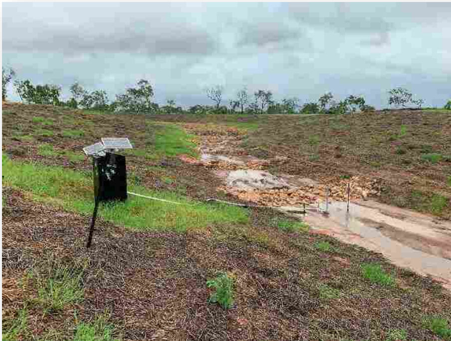
Plate 15 Porous check dams installed in the bed of Treatment 3.
