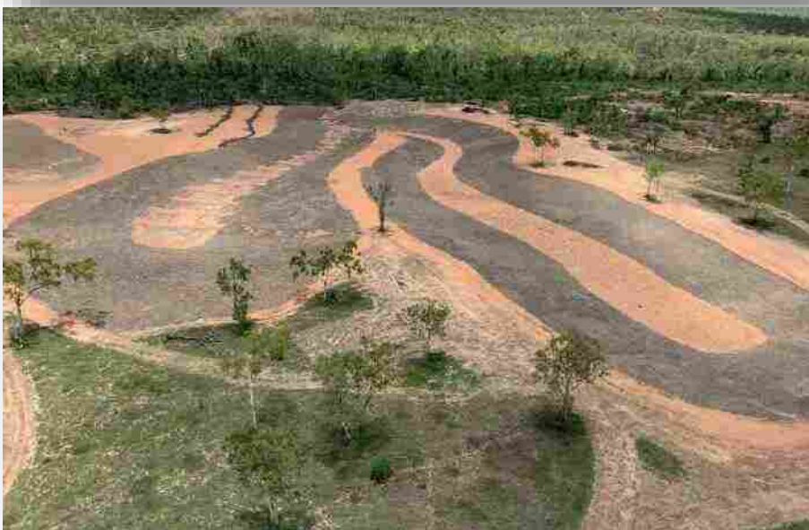
Plate 8 Treatment areas 3 and 4 post remediation in December 2018.
