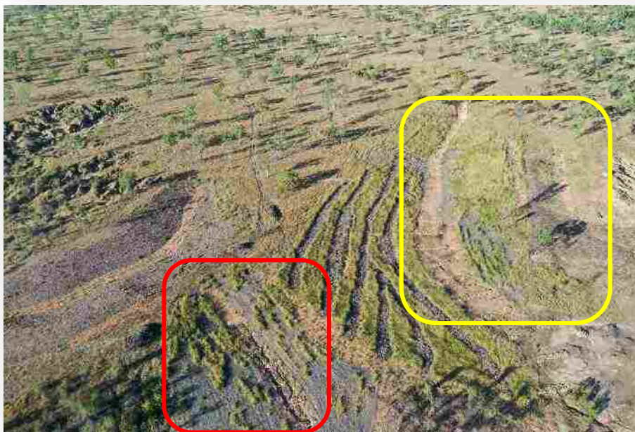
Plate 24 Areas of bagasse spreading on the Treatment 8 and 8b batters, yellow rectangle indicates areas where a mulch blower was utilised, red rectangle is where a side-tipper and grader were used.
