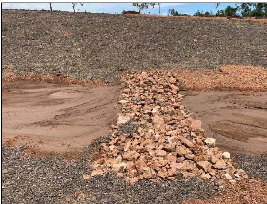
Plate 10 Approximately 200mm depth of sediment deposition behind porous check dams in Treatment 3, creating the typical stepped profile (flow from photo left to right)
