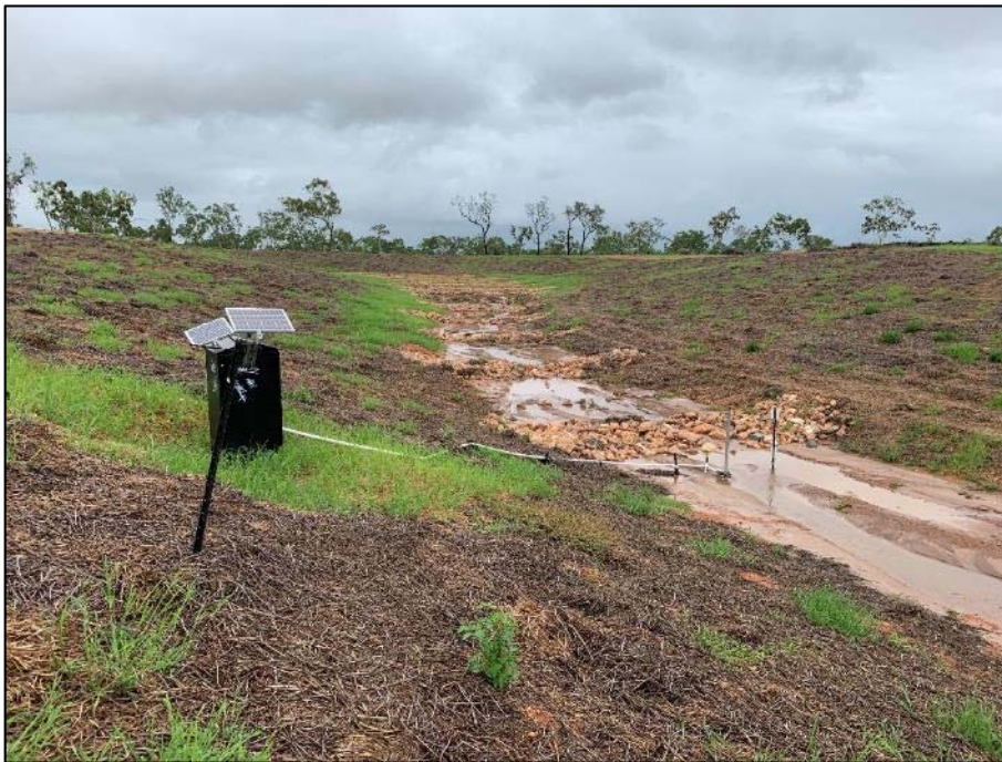
Plate 9 Porous check dams installed in the bed of Treatment 3.
