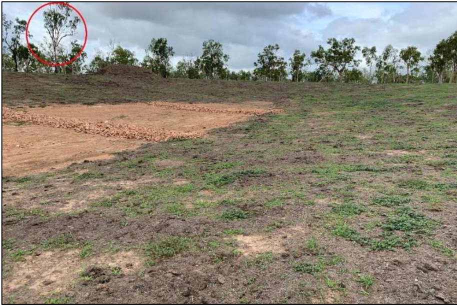
Plate 14 Treatment 7 three months after construction in December 2018
