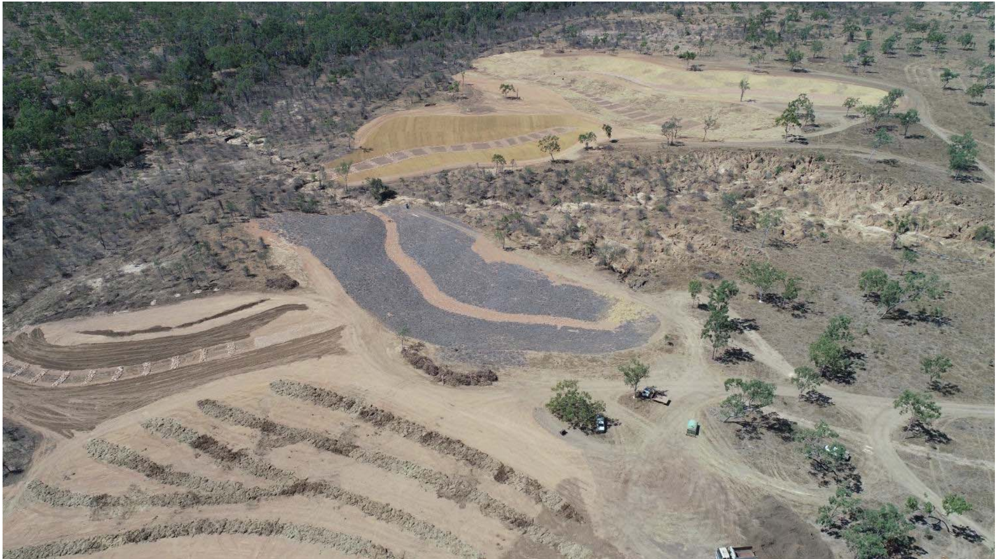
Plate 2 Innovative Gully Remediation Project works underway in 2018 – Strathalbyn Station
