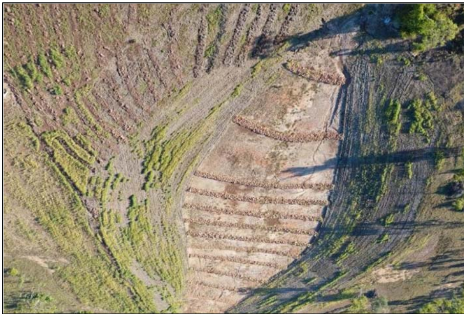
Plate 11 Outflanking of check dams at the downstream end of Treatment 6
