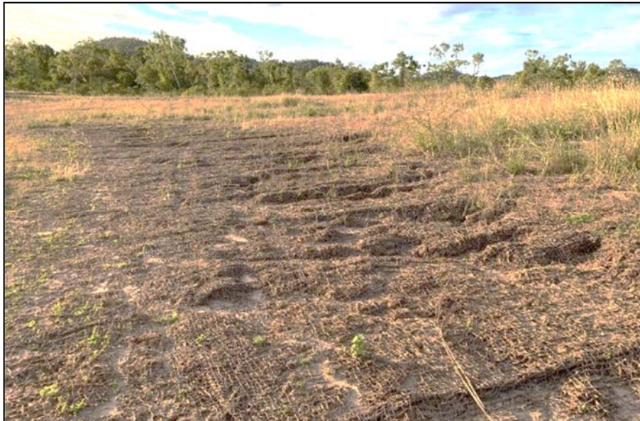
Plate 13 Rill erosion underneath the jute mesh covers installed on the Treatment 2 batters
