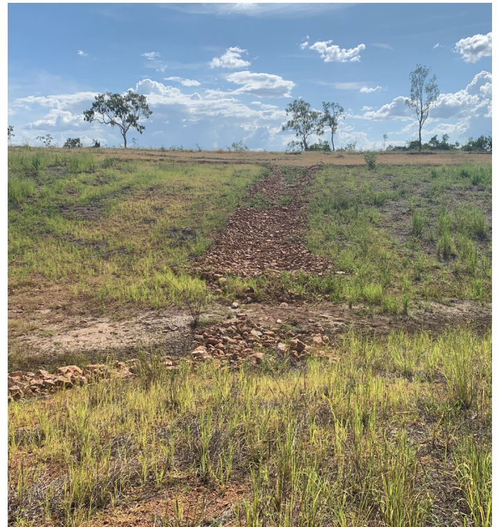
Batter repair using diversion bunds and a batter chute (left image 2019, right image 2020). Photo credits: Fruition Environmental Pty Ltd 2020
