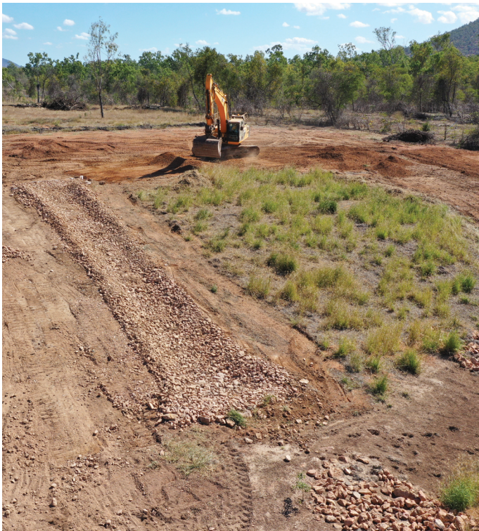
Batter repair using diversion bunds and a batter chute (left image 2019, right image 2020). Photo credits: Fruition Environmental Pty Ltd 2020
