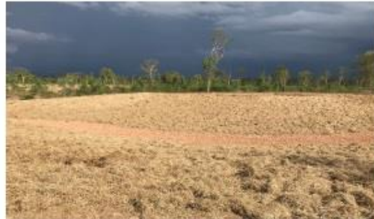
Remediation works were tricky in the late dry/early wet, but the job was completed on time.
