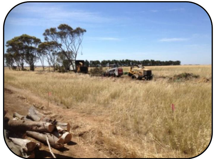
Removing the trees from site
