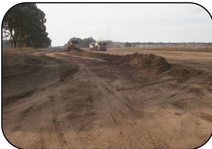
The site being scraped
