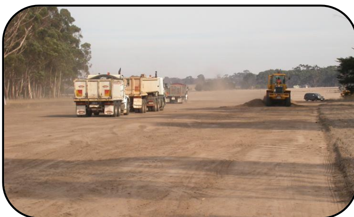
The topsoil being removed and carted offsite
