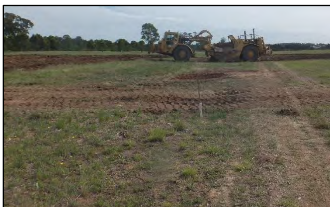
Image 5. Wayne in his large scalper starts laying topsoil in spoil zone at Bungarribee.
