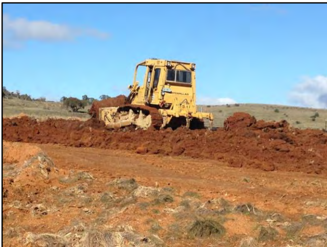
Apple Box patch, site preparation, April 2014
