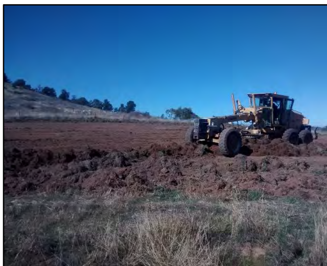
Barrer: Site preparation and inverting the soil profile April 2015.
